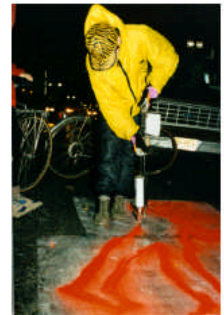
Stenciling in progress
